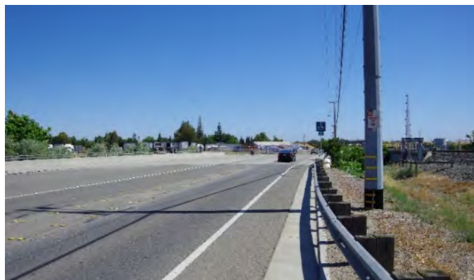
Photo 4-6: Atkinson Street Bridge over Dry Creek, looking north
