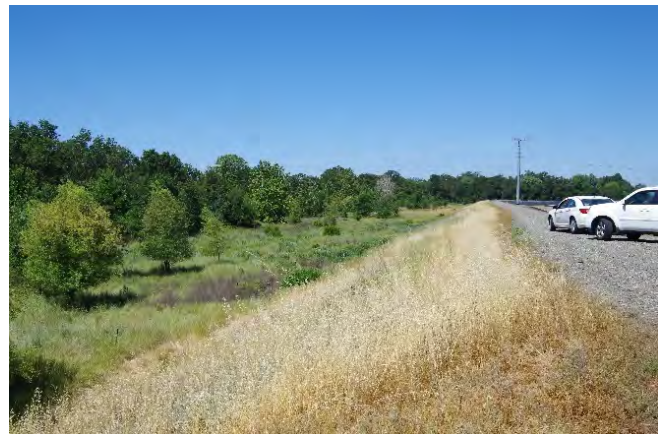
Photo 4-4: New levee at Roseville WWTP, looking west.
