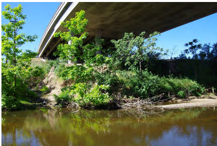
Photo 4-8: Location of potential trail at south end of Foothills Boulevard Bridge.
