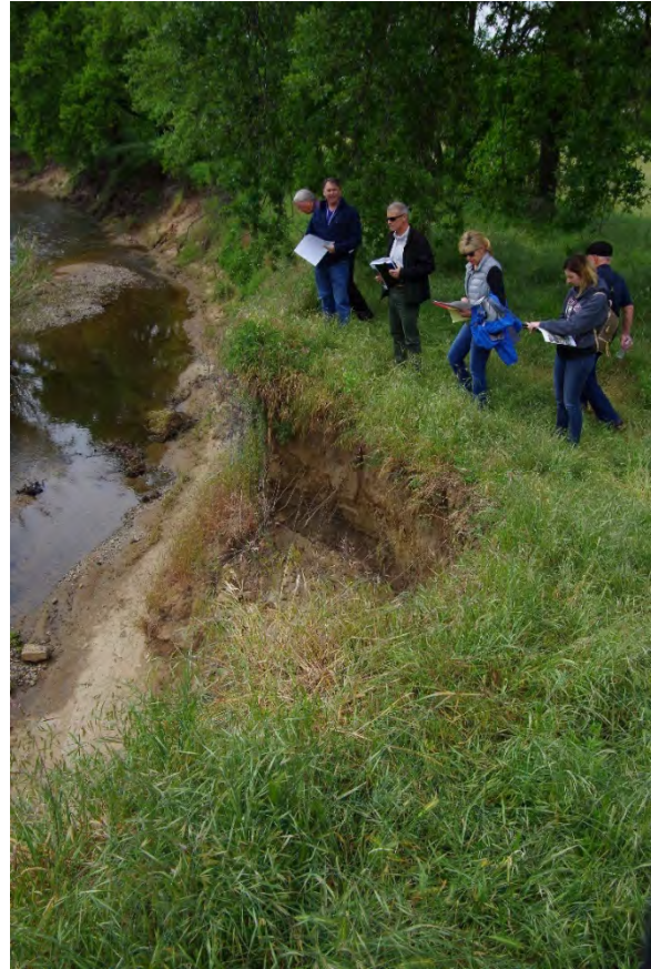
Photo 4-1: Site walk with property owner.
